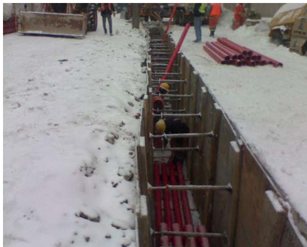
Figure 18 Duct Line Under Construction
