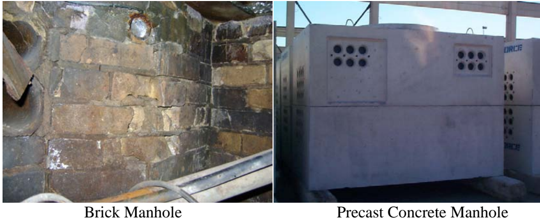
Figure 13 Manhole Installations
