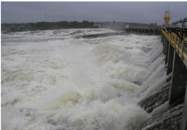
Photo 5: Turbulence downstream of spillway bays 45 - 65; spilling through bays 47, 49-52 and 56-65.
