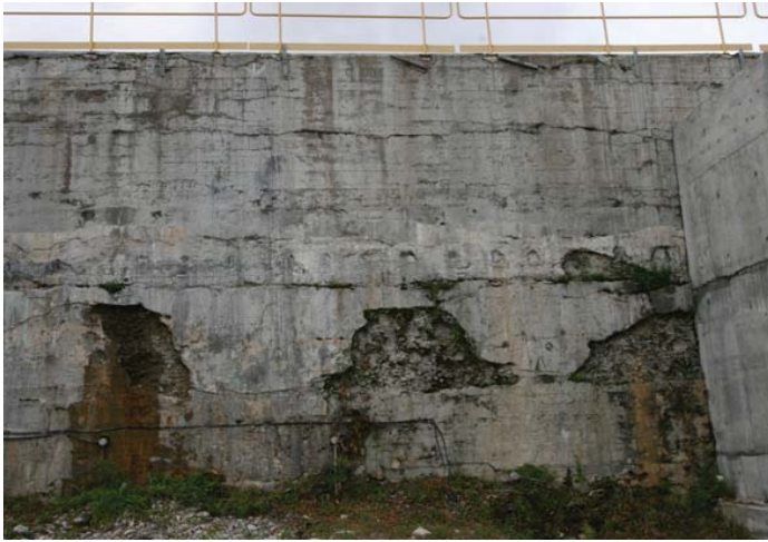
Photo 7: Concrete spalls along downstream north end of east gravity dam; leakage is evident through cracks (typical).
