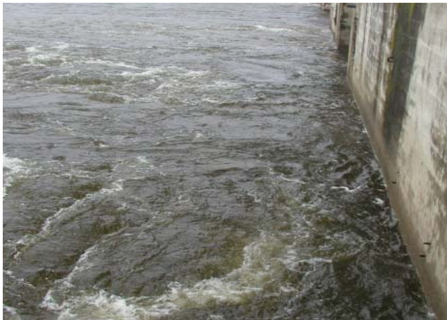
Photo 3: Turbulence at powerhouse tailrace
