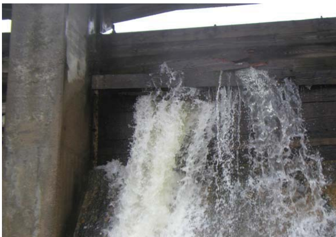
Photos 11 & 12: Stoplogs are damaged in the curved spillway bay 112, due to high ice flow in spring, as noted during the spring inspection. Damage and leakage appears to have increased.
