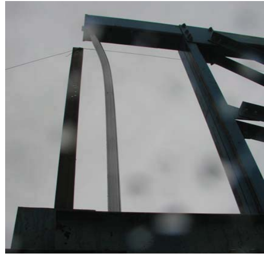
Photo 8: Hoist at spillway bay 36, was damaged in high winds.
