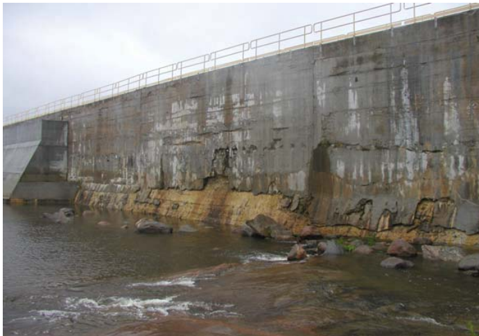
Photos 9 & 10: Concrete spill and leakage at block 19; concrete is offset to 75 mm.
