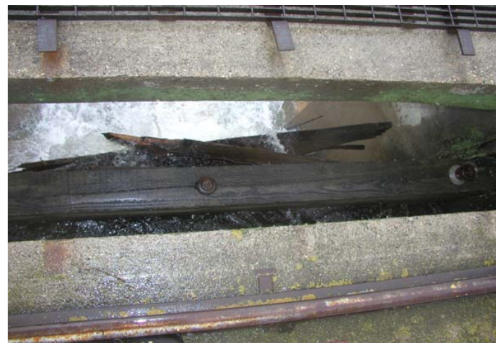
Photos 11 & 12: Stoplogs are damaged in the curved spillway bay 112, due to high ice flow in spring, as noted during the spring inspection. Damage and leakage appears to have increased.
