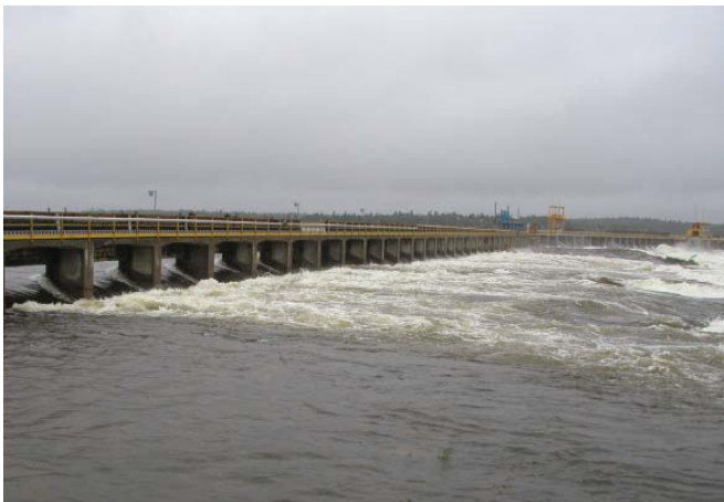
Photo 1: General downstream view of spillways and sluiceways.
