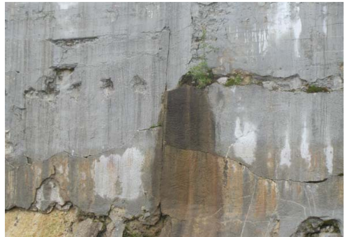
Photos 9 & 10: Concrete spill and leakage at block 19; concrete is offset to 75 mm.
