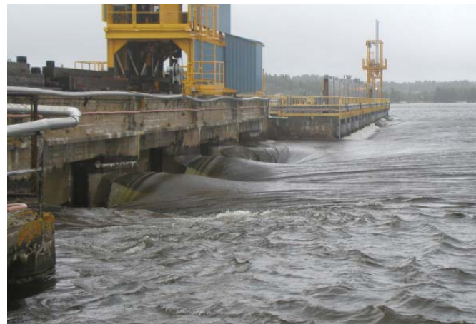
Photo 6: Upstream sluiceway, spilling through openings 2, 3 and 4.
