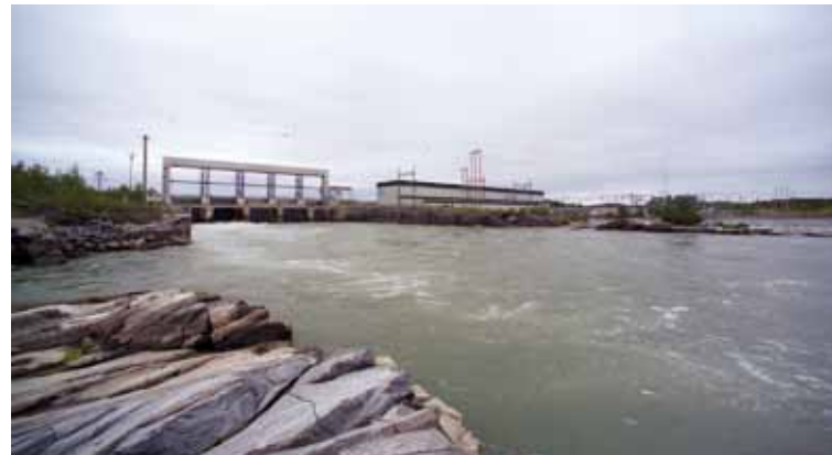
Manitoba Hydro's Jenpeg Generating Station on the Upper Nelson River.
