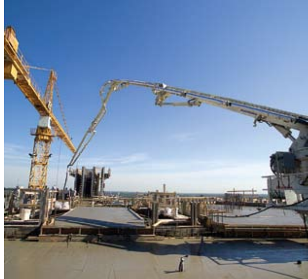
Topping off: Pouring concrete on the building's 22nd floor.
