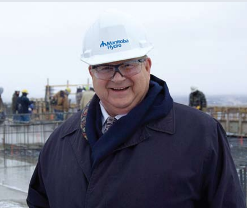
President and CEO Bob Brennan at the ceremony announcing the completion of concrete placement on the 22nd floor—a milestone construction event.
