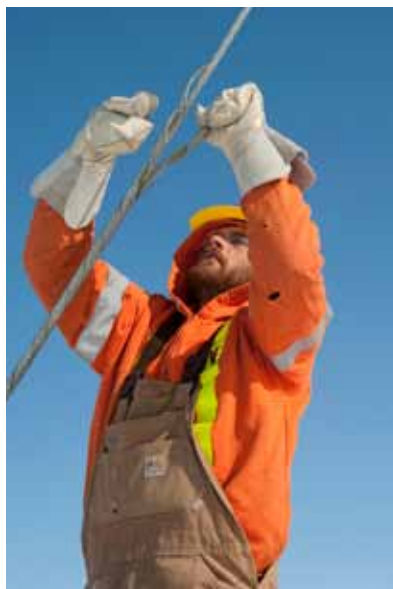
Left: One of the towers on the new Wuskwatim transmission line is lifted into place. Centre: Mitch Kula, of Valard Construction, tensions a guy wire to stabilize the tower. Right: Digging a trench for a natural gas transmission pipeline.
