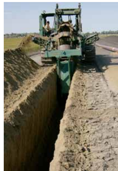
Left: One of the towers on the new Wuskwatim transmission line is lifted into place. Centre: Mitch Kula, of Valard Construction, tensions a guy wire to stabilize the tower. Right: Digging a trench for a natural gas transmission pipeline.
