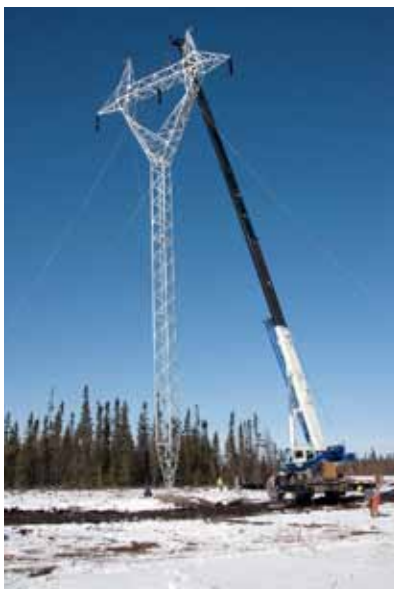
Left: One of the towers on the new Wuskwatim transmission line is lifted into place. Centre: Mitch Kula, of Valard Construction, tensions a guy wire to stabilize the tower. Right: Digging a trench for a natural gas transmission pipeline.
