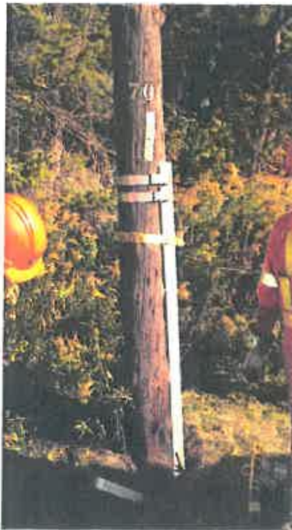
Figure 2: Pole Reinforcement Installation
