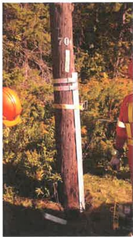
Figure 2: Pole Reinforcement Installation
