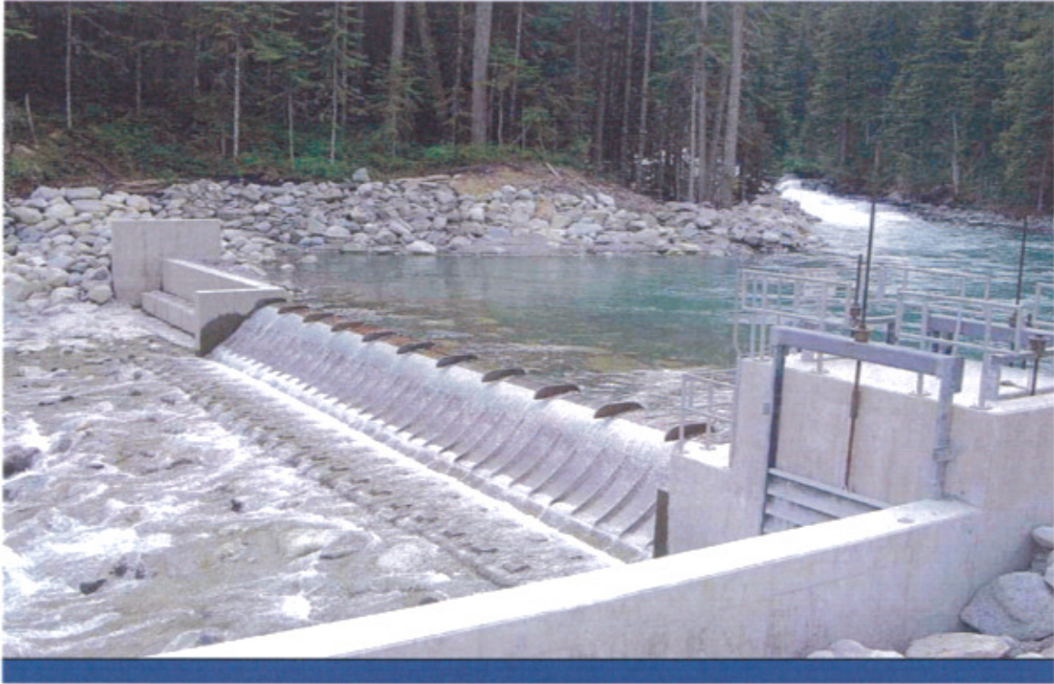
Brandywine Creek - Fish Friendly Intake Weir
