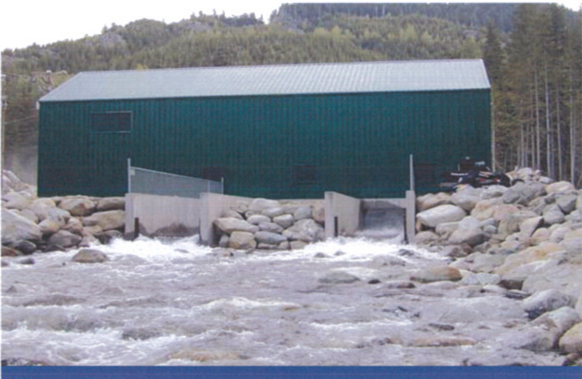
Brandywine Creek - Powerhouse
