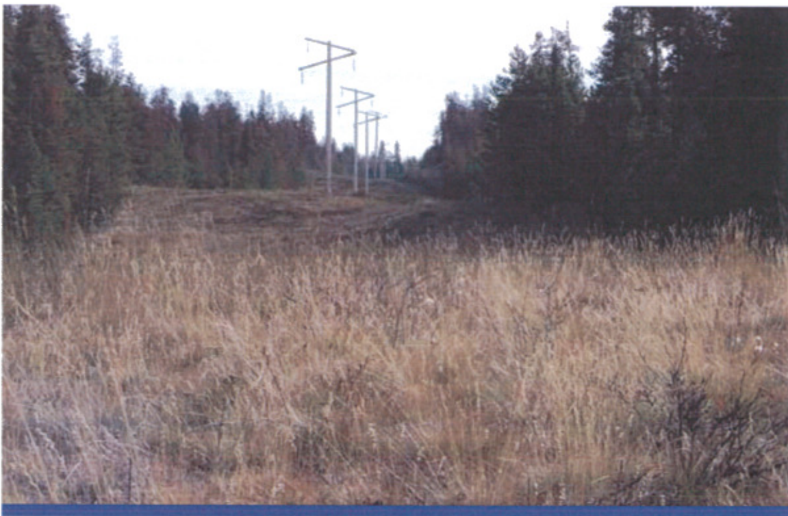
Typical Transmission Line
