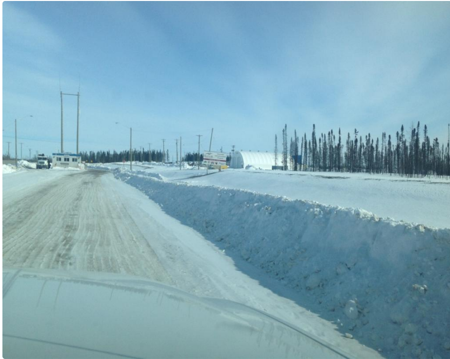
Gated entrance to Keeyask Infrastructure Project
