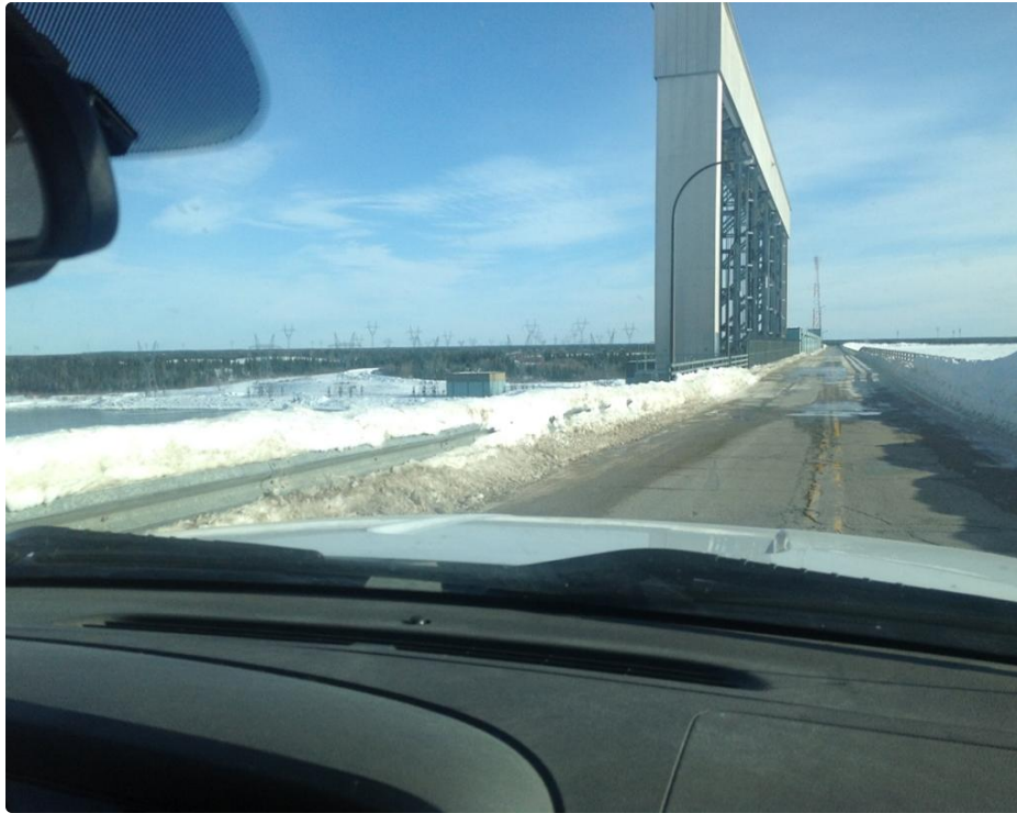
Long Spruce Dam
