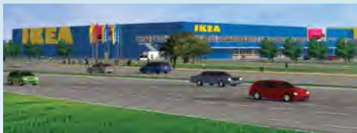
The IKEA building is heated and cooled by one of the largest geothermal systems in Manitoba.
