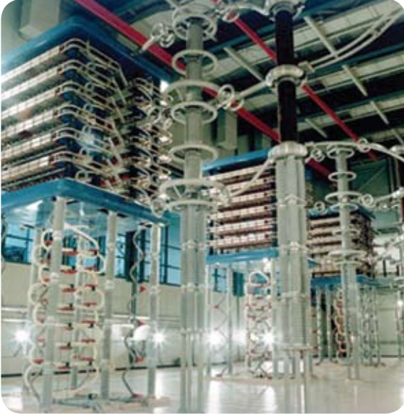
Figure 25.2: A valve hall from Valve Group VG13 of the Nelson River project in Canada, showing the large developed length used for the coolant pipework to span the distance between earth and the base of the valve stack at 330 kVDC.
