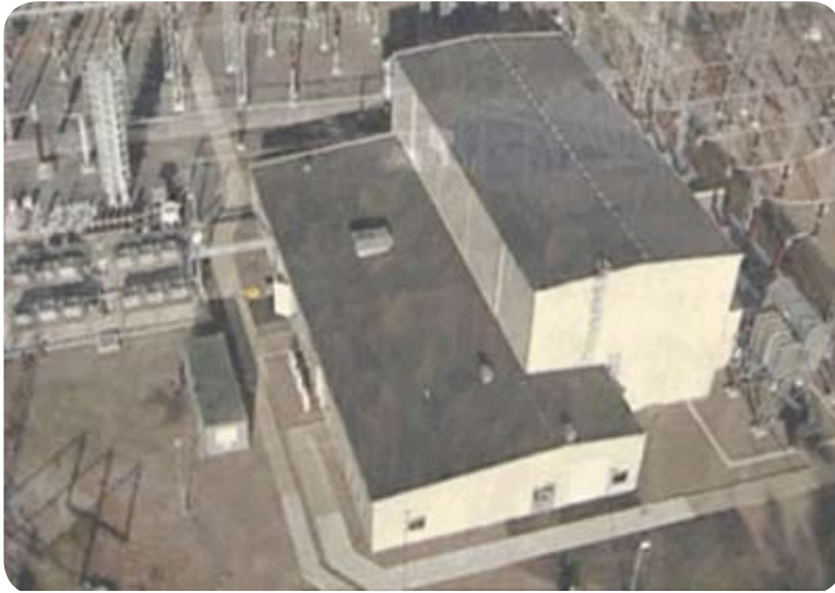
Figure 5.2: Lindome, Sweden, Converter Station; Part of the 380 MW KontiSkan HVDC Interconnection
