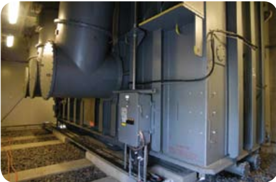
Converter Transformers
