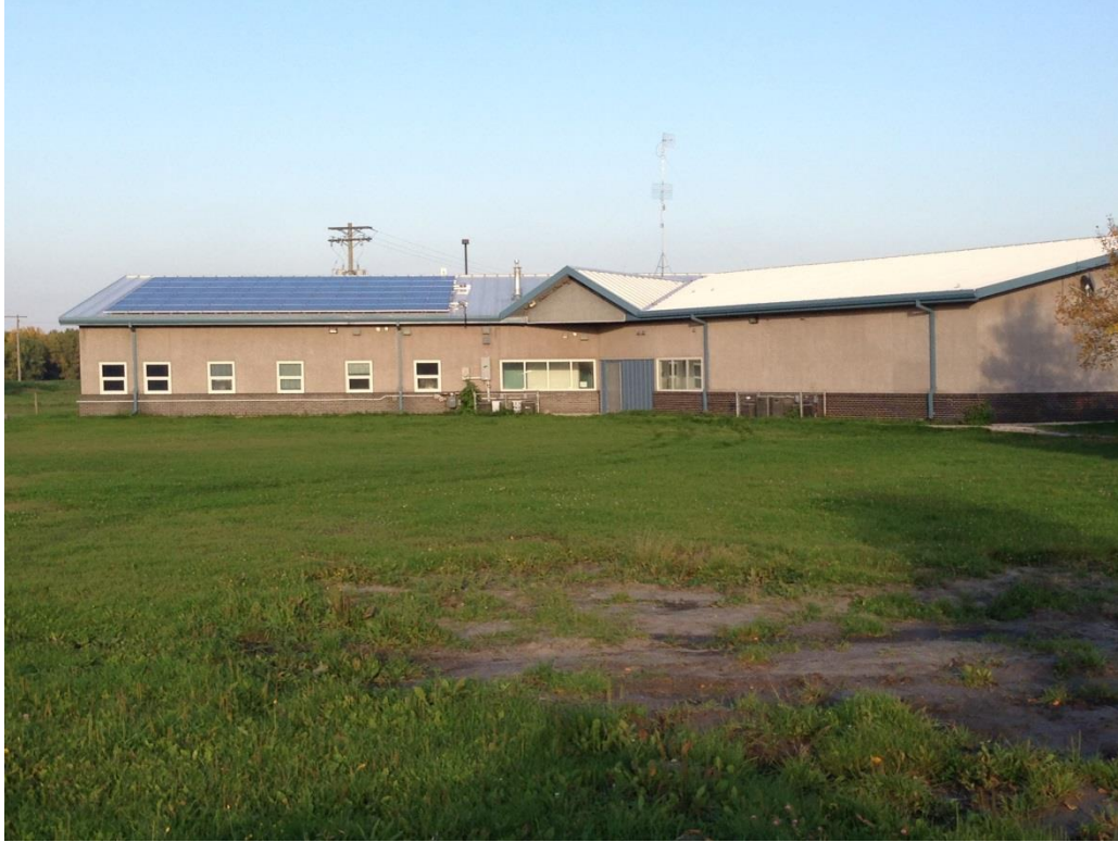
Figure 4: Administrative building in Portage la Prairie with 21 kW of solar panels (courtesy of Solar Solutions Inc.)
