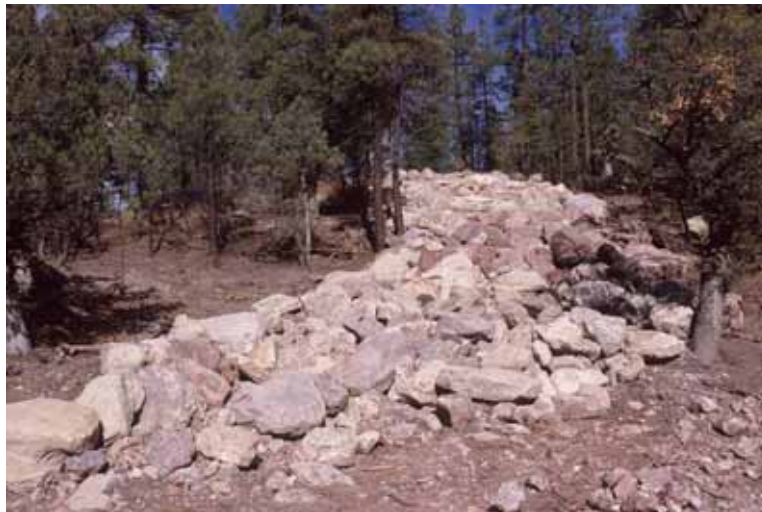
Figure 55. Photo. Large boulders pPlaced in the right of way as a barrier to elk and deer along State Route 260 in Arizona (copyright: Marcel Huijser).
