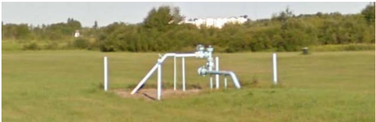
End of NPS 6 line at Swan River Town Border Station Take-Off
